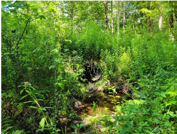
Downstream Crown Point Road Culvert
