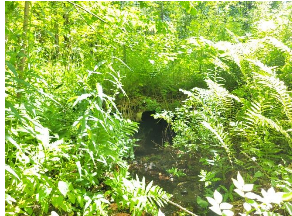
Upstream Crown Point Road Culvert
